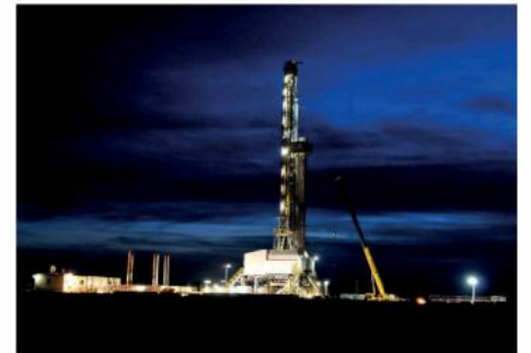
WEST NEWTON - NIGHTTIME OPERATIONS
